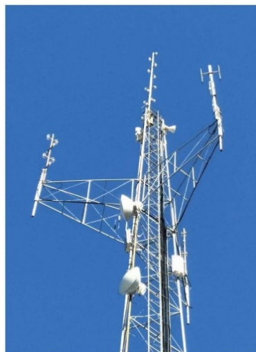
ATV quads on the tower
